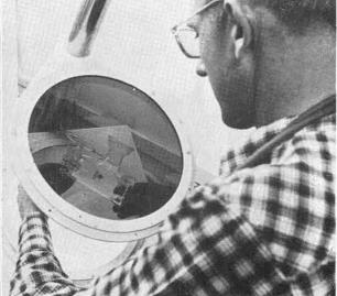
in the glass. Operator Charlie DeMoss, in picture at right, examines glass apparatus under a polariascope which reveals internal stresses or strains remaining after work on the glass is completed.
